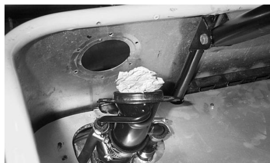
Figure 184: Old filler boss removed
